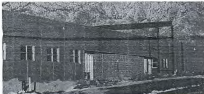
New Command Center is nearing completion at Eubank & Holly NE.
