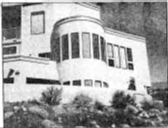
Tamara is putting in a river rock path to divert water away from the Griffin manse.
