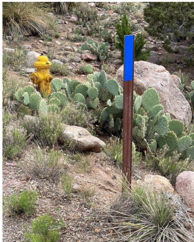
Example of a blue reflector stake marking the location of a fire hydrant
