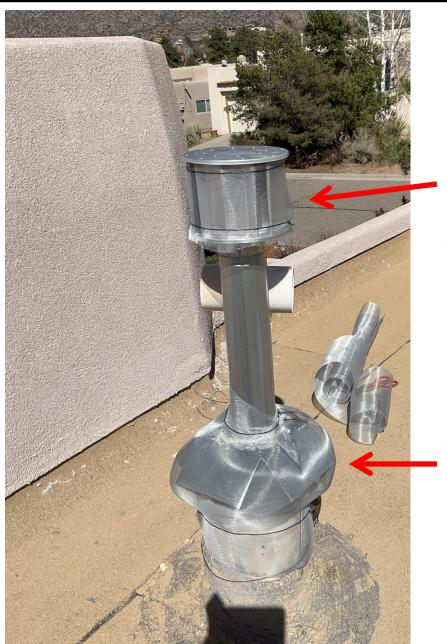
Strip of wire mesh around chimney exhaust held in place with twisted black wire.
