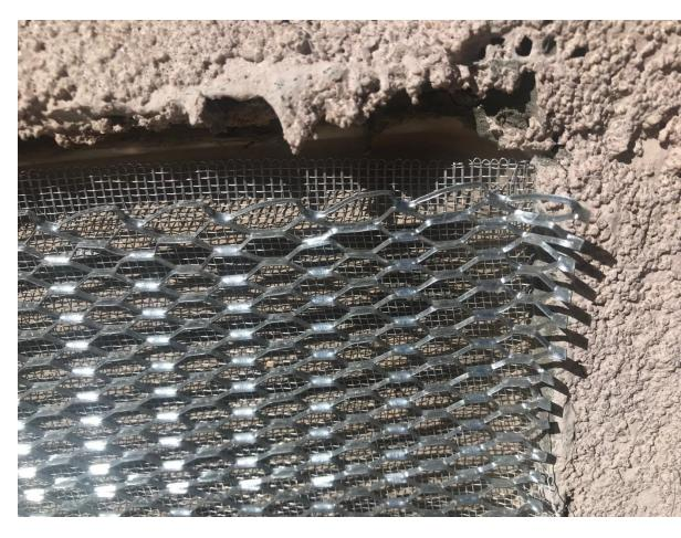
If the louvered cover can be removed without damaging stucco, the Plaster Lath may not be needed. Wrap the oversized wire mesh (cut 1-inch wider than the louvered cover on all 4 sides) around the cover and replace.
