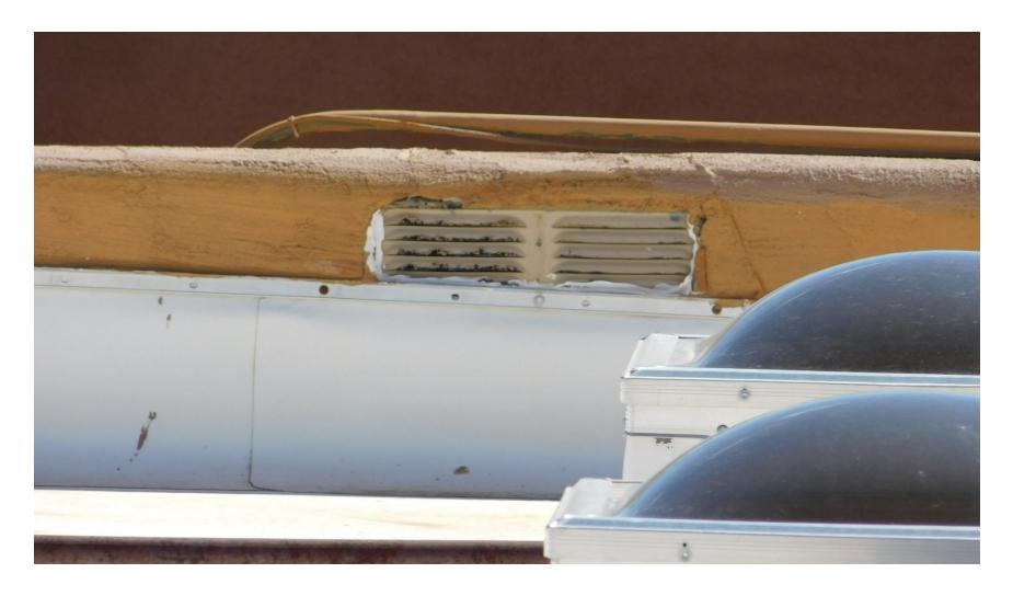
These vent covers were installed with louvers up which could scoop RAIN or EMBERS inside the walls.
