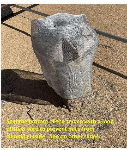
Secure the screen with black wire OR sheet metal screws into the original vent housing. Oversize screening to improve air flow.
