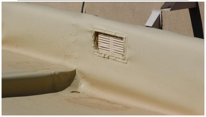
Typical roof vent. Notice the bent louvers which will admit larger particles.
