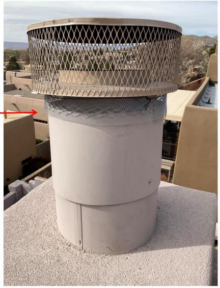
IF your fireplace doesn't have a damper OR sealed doors, consider screening the upper vent OR installing a different chimney hood. The path from the firebox to the outside should not allow embers to flow down inside your home.
